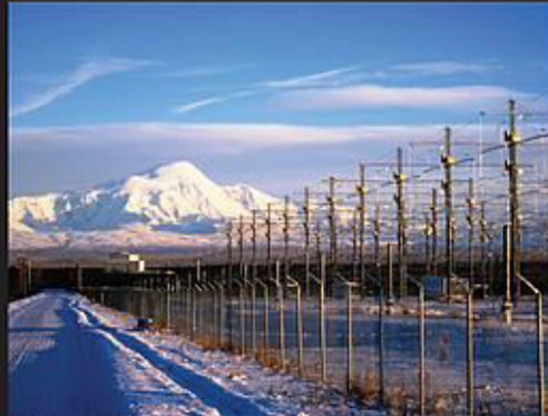
The massively powerful HAARP ionosphere heater transmission facility in Alaska.
